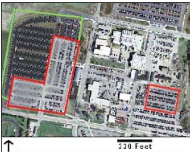
URI's permeable parking lots - The two original permeable asphalt parking lots built in 2002 and 2003 are outlined in red. The 2005 parking lot extension is outlined in green.
