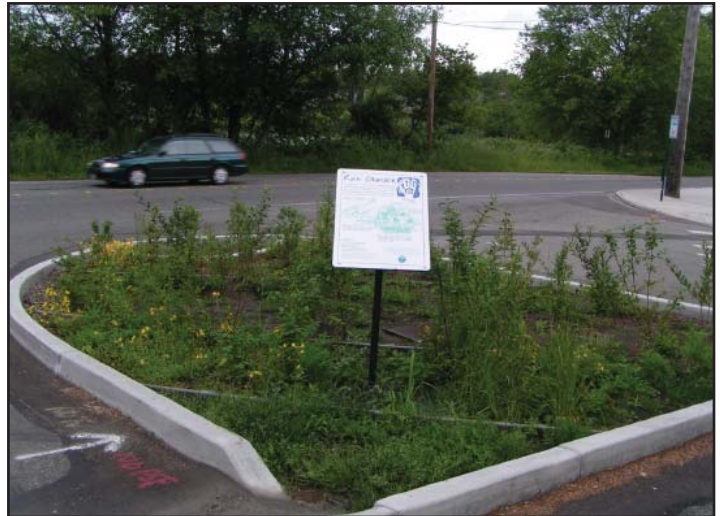
The raingarden in Bloedel Donovan Park helps protect the water quality in nearby Lake Whatcom, and recharge groundwater supplies.
