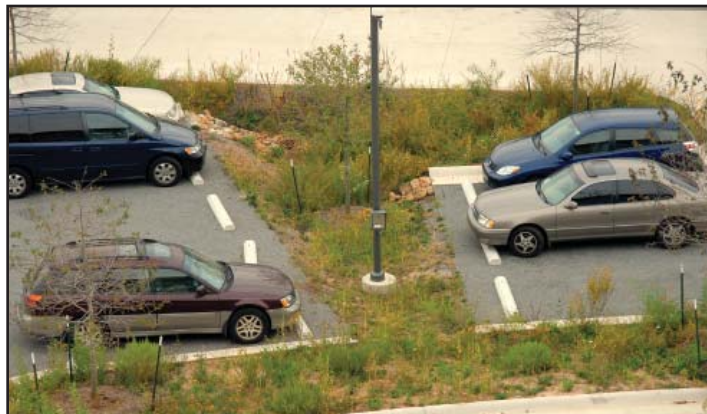
Strategically sloped vegetated strips are a better option than conventional grassy parking islands for collecting and filtering runoff.
