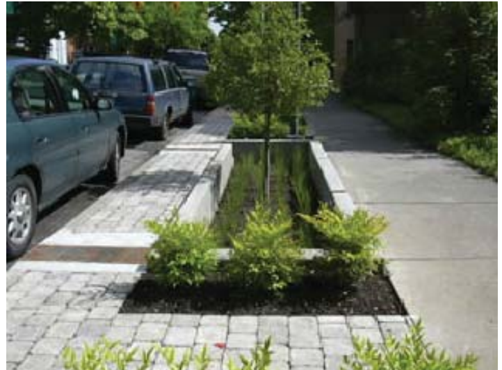
One of many rain gardens being built throughout Portland as part of the city's Green Streets program.
