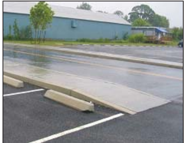
Rainwater infiltrates the porous asphalt (left), but accumulates on adjacent road paved with conventional material (right).
